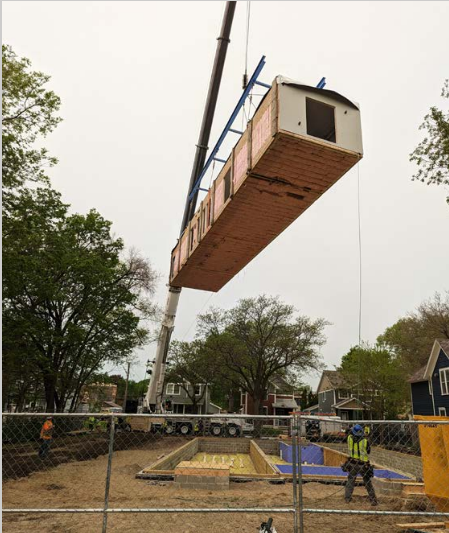
A module being craned onto its site in Minneapolis. (Courtesy DJR)
