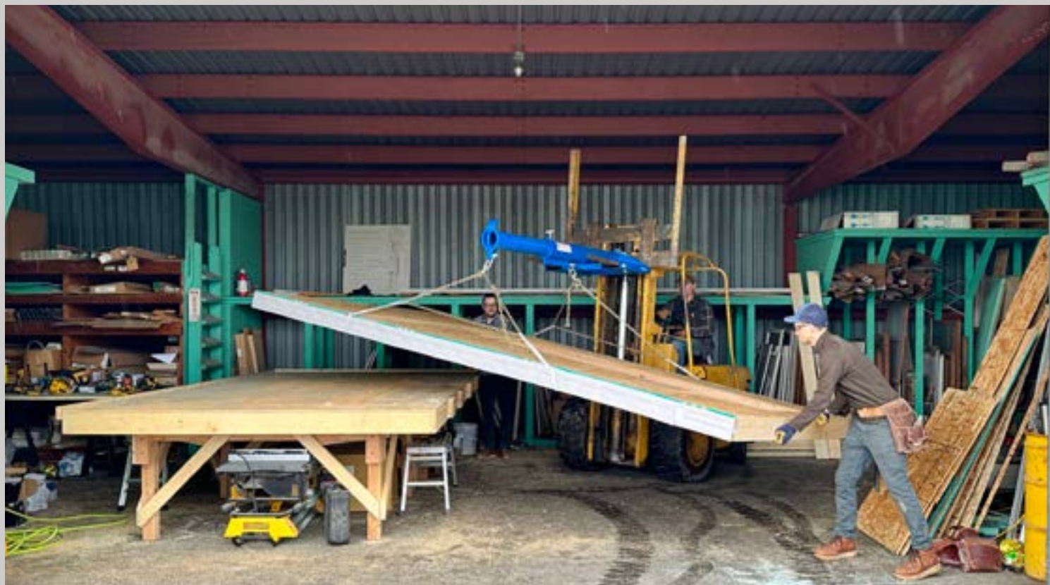
Panels being manufactured at Lagom Modular's facility in Minnesota. (Courtesy Lagom Modular)
