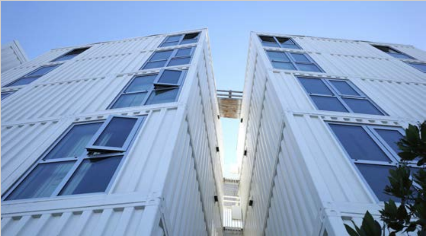
Each one-bedroom unit at Isla Intersections is composed of three container modules.
