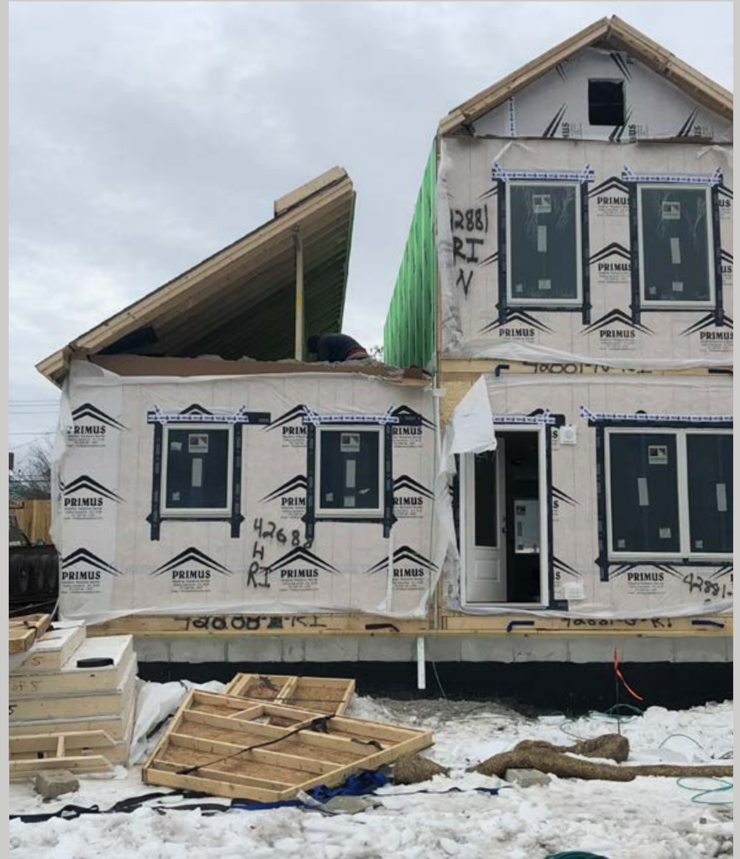
Flat-packed roofs were folded upward into place after on-site module assembly. (Courtesy Truth Box Architects)
