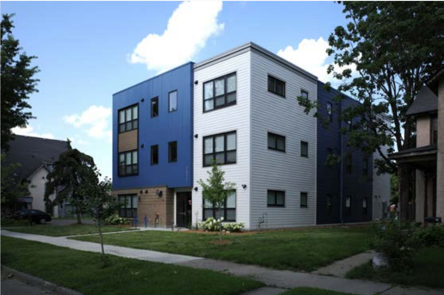
A six-unit apartment building constructed from nine volumetric modules in Minneapolis, Minnesota.
