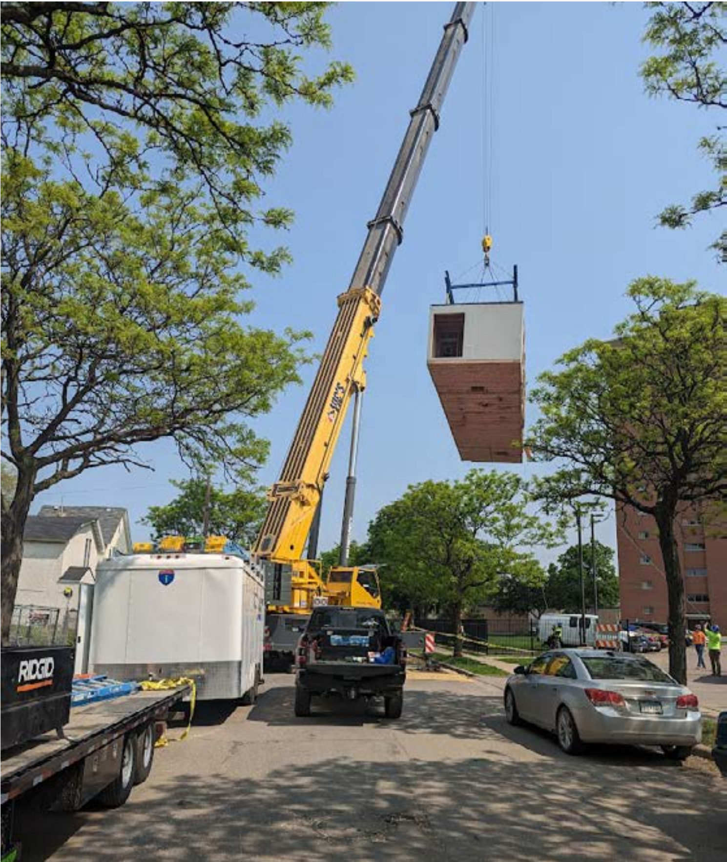
A volumetric module being lifted into place on one of the MPHA’s sites in Minneapolis, Minnesota. (Courtesy DJR)
