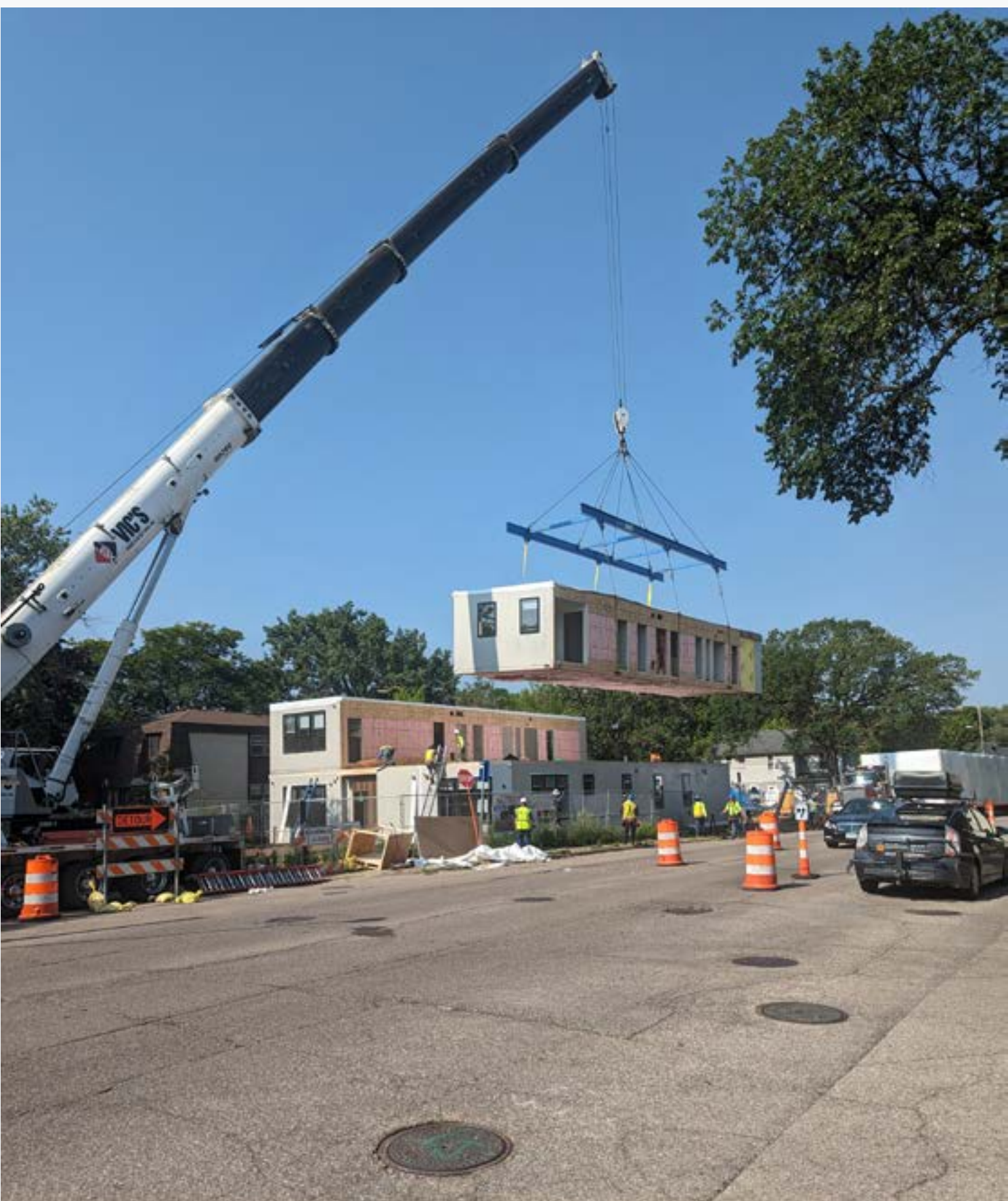
The MPHA's buildings were assembled one by one, with crews moving from site to site over several weeks. (Courtesy DJR)
