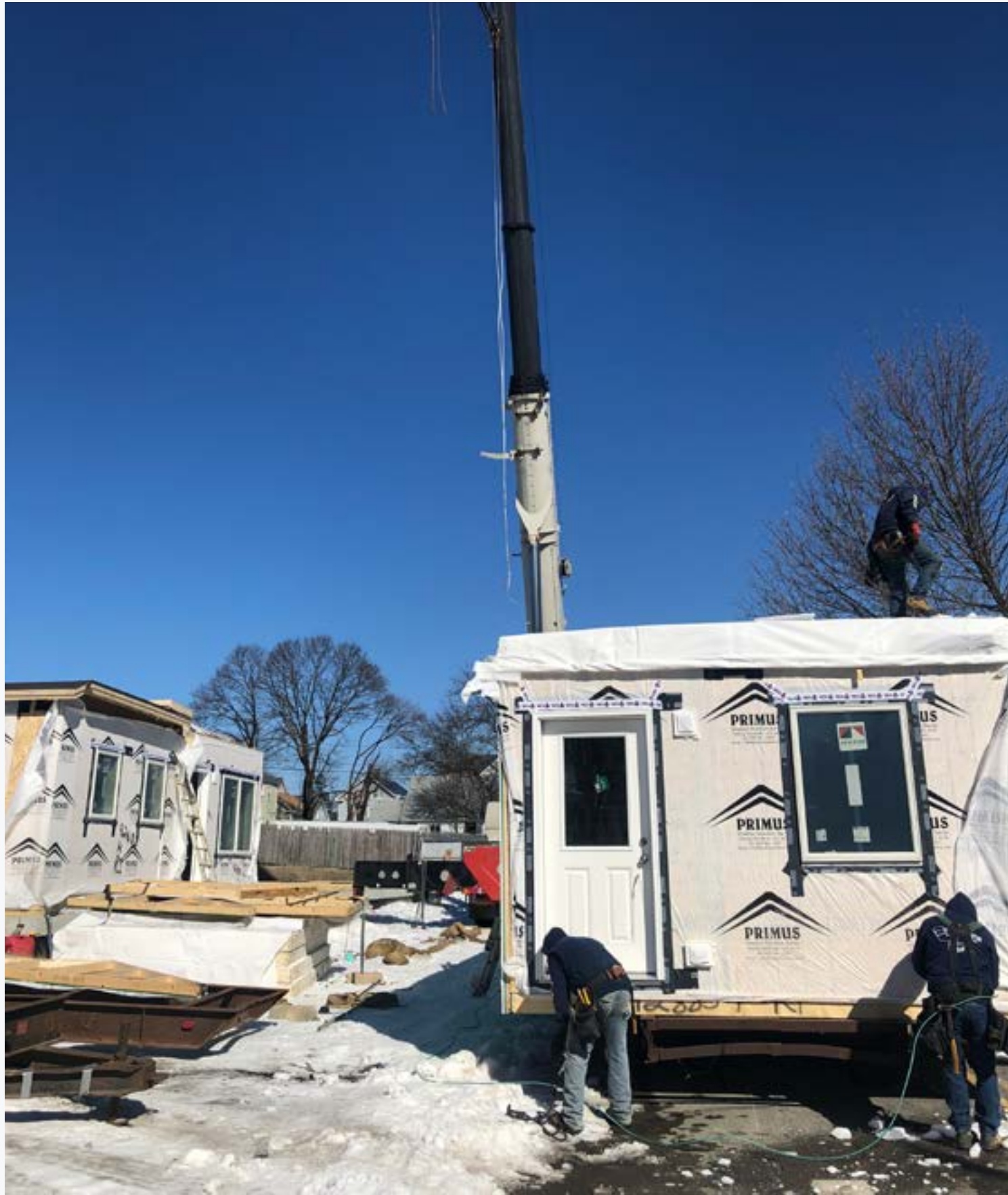
Crews prepare to hoist a volumetric module onto the site of the Bowdoin Street Rowhouse. (Courtesy Truth Box Architects)
