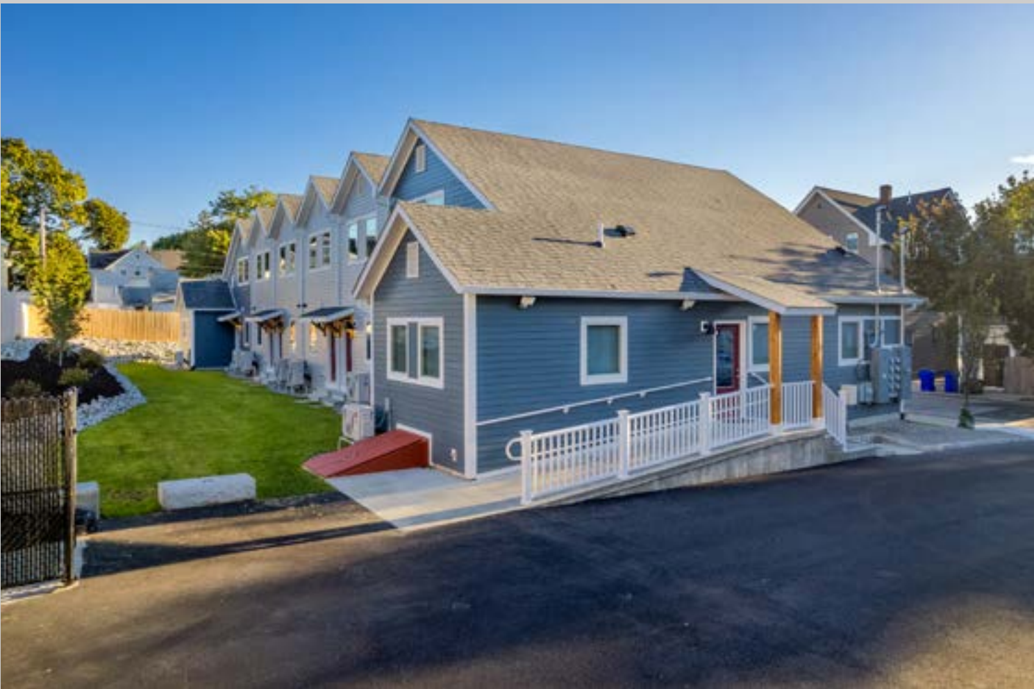
Single-story units on either end continue the same roof pitch as the duplexes. (Jason Wessel Photography)
