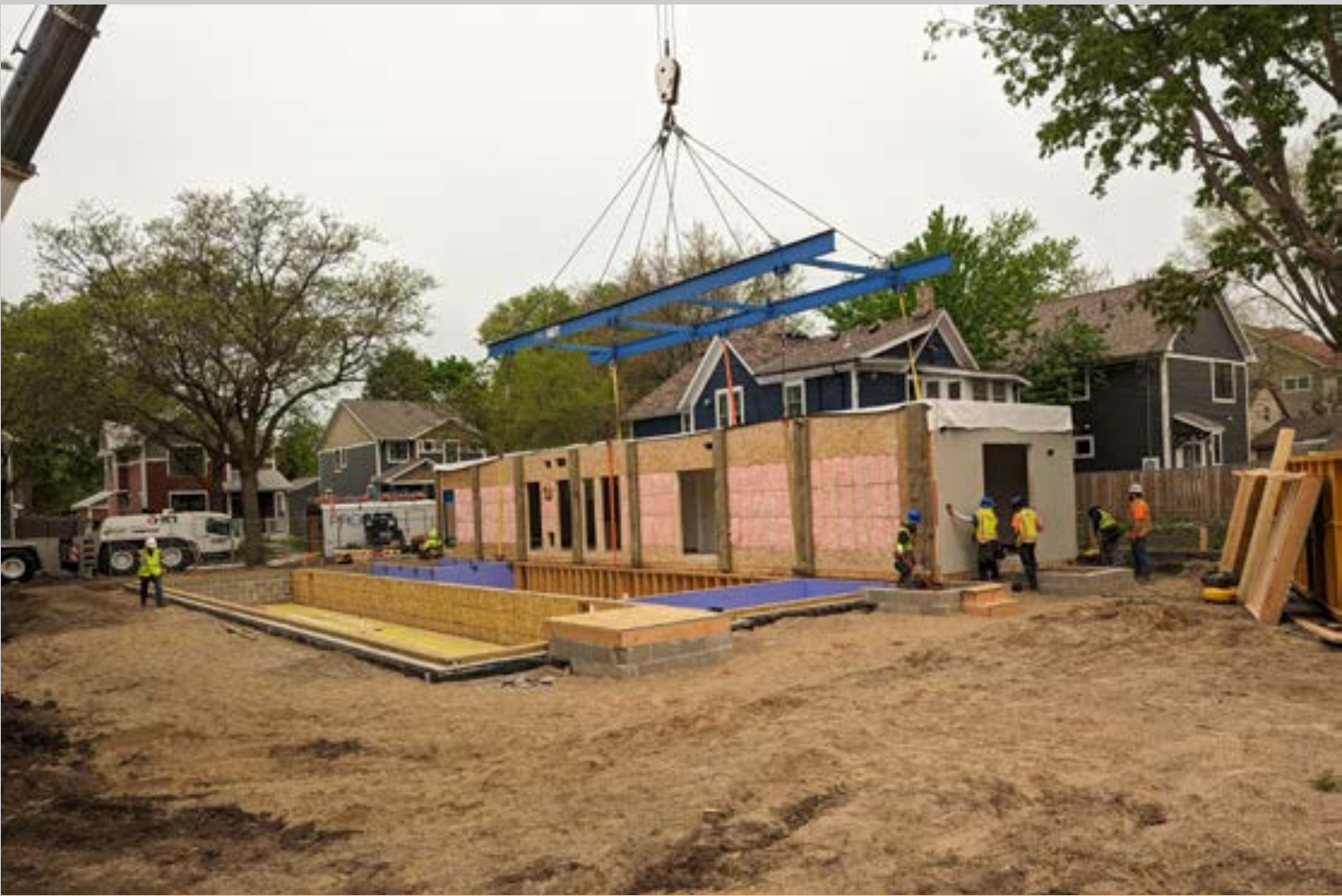
Workers set a single volumetric module on the foundation of one of MPHA’s scattered site buildings. (Courtesy DJR)
