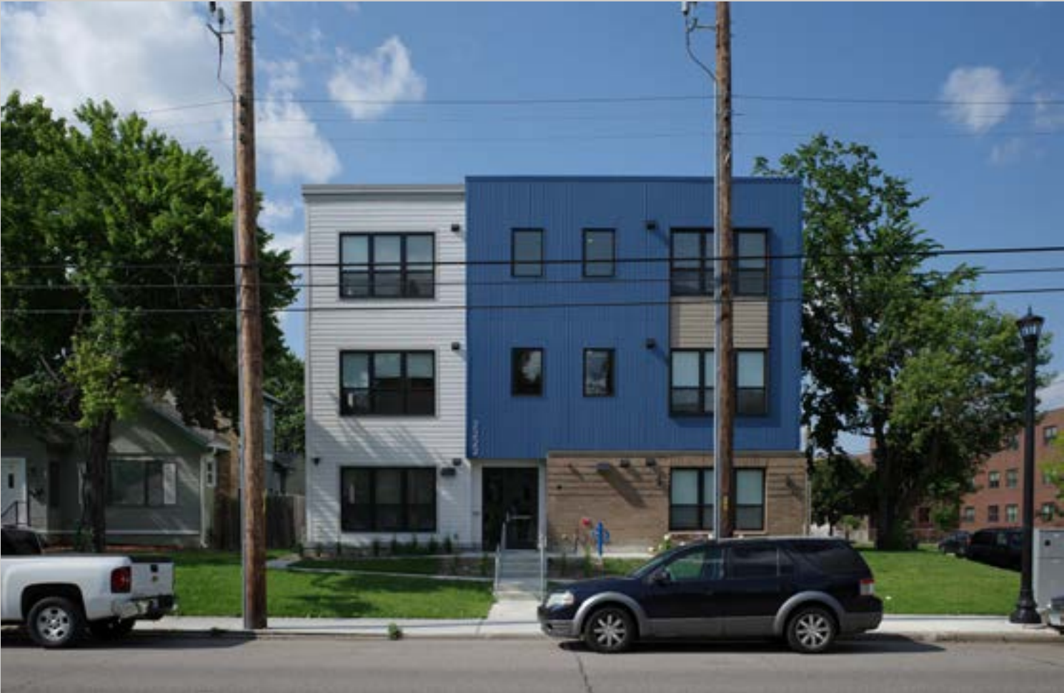
A six-unit apartment building constructed from nine volumetric modules in Minneapolis, Minnesota.
