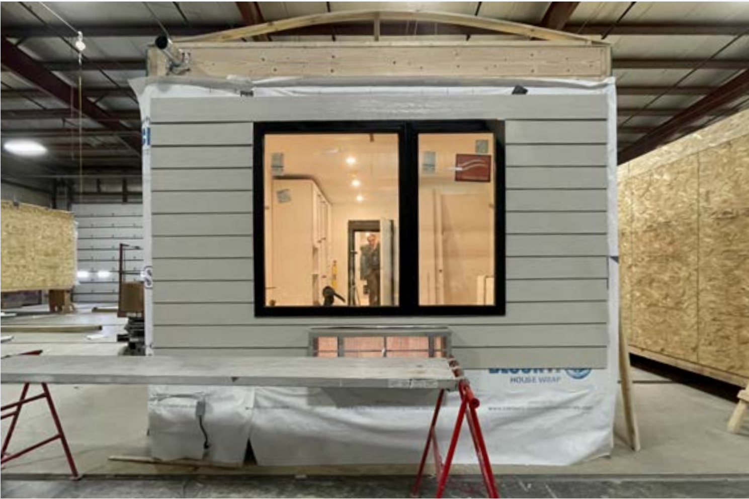
Plover Place's 3-D modules were fitted with siding, windows, and millwork before shipment to site. (Courtesy One Roof)
