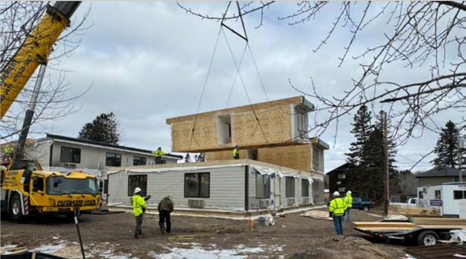
Plover Place’s modules being craned into place. (Courtesy One Roof)
