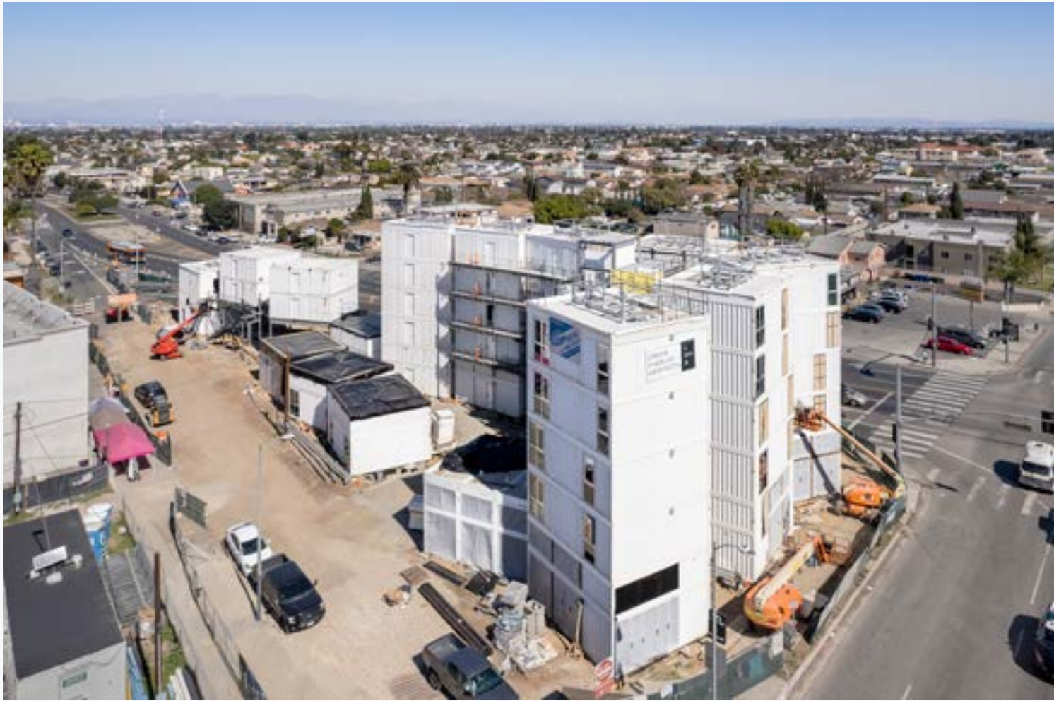
Isla Intersections' massing consists of several towers of modules stacked to varying heights. (Paul Vu, courtesy LOHA)
