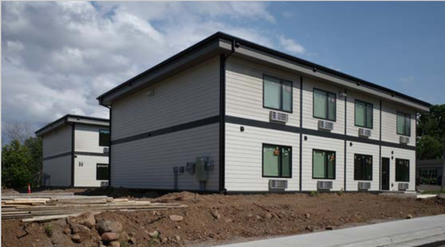
Plover Place consists of two identical buildings built from eight volumetric modules each.
